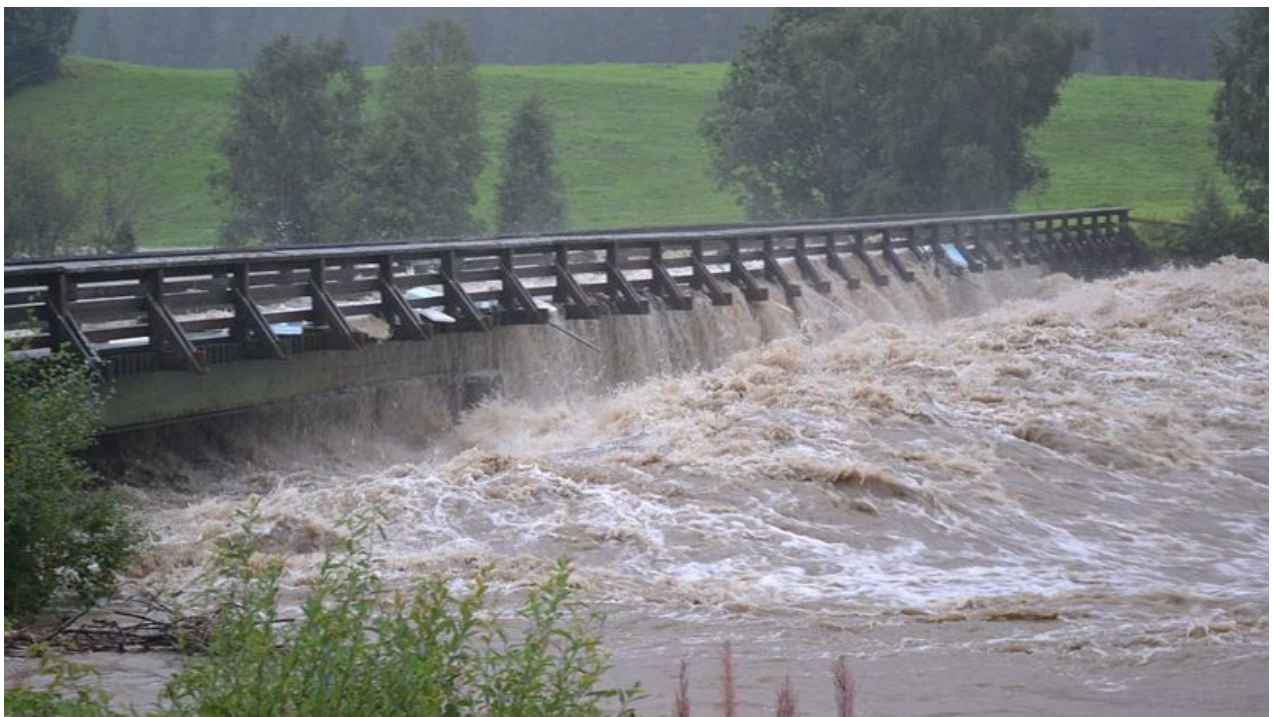
Extreme precipitation leads to flooding at Bollingmo bridge, Holtålen, August 2011
