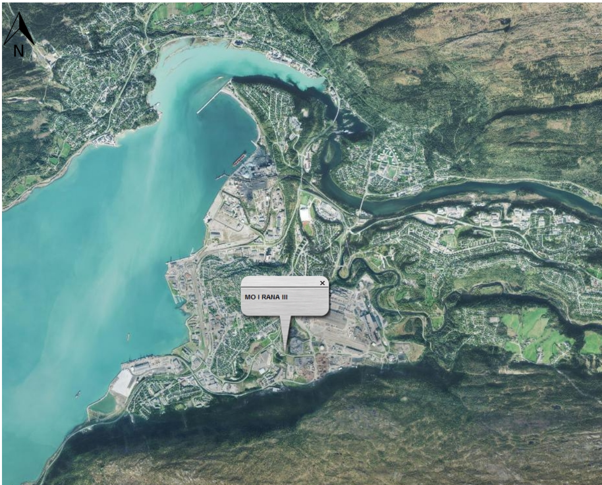
Figure 17: Aerial photo from Mo i Rana met. station near the town center and Ranfjorden.
