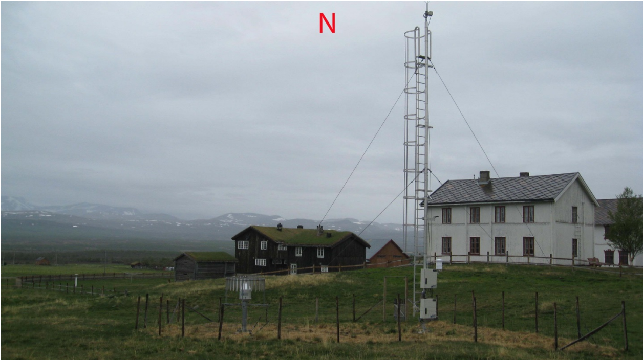
Weather station towards North
