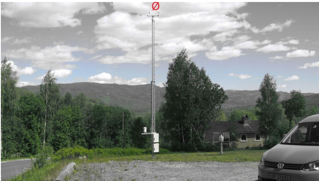
Weather station towards East
