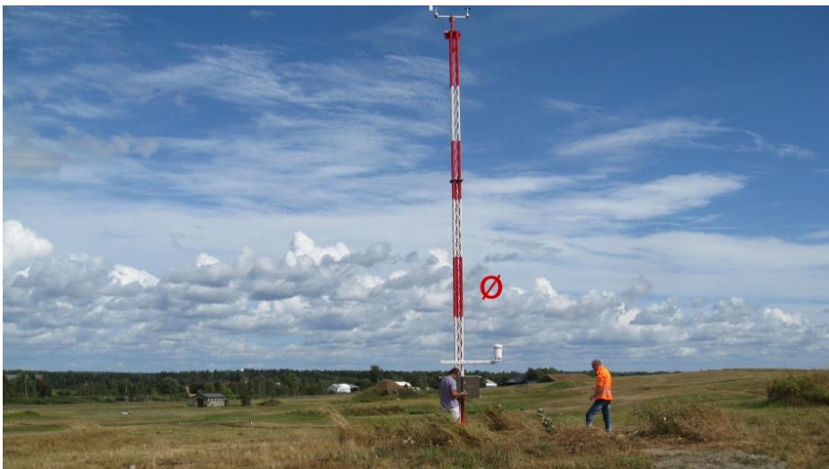
Figure 21: Rygge airport weather station. Photo: MET Norway
