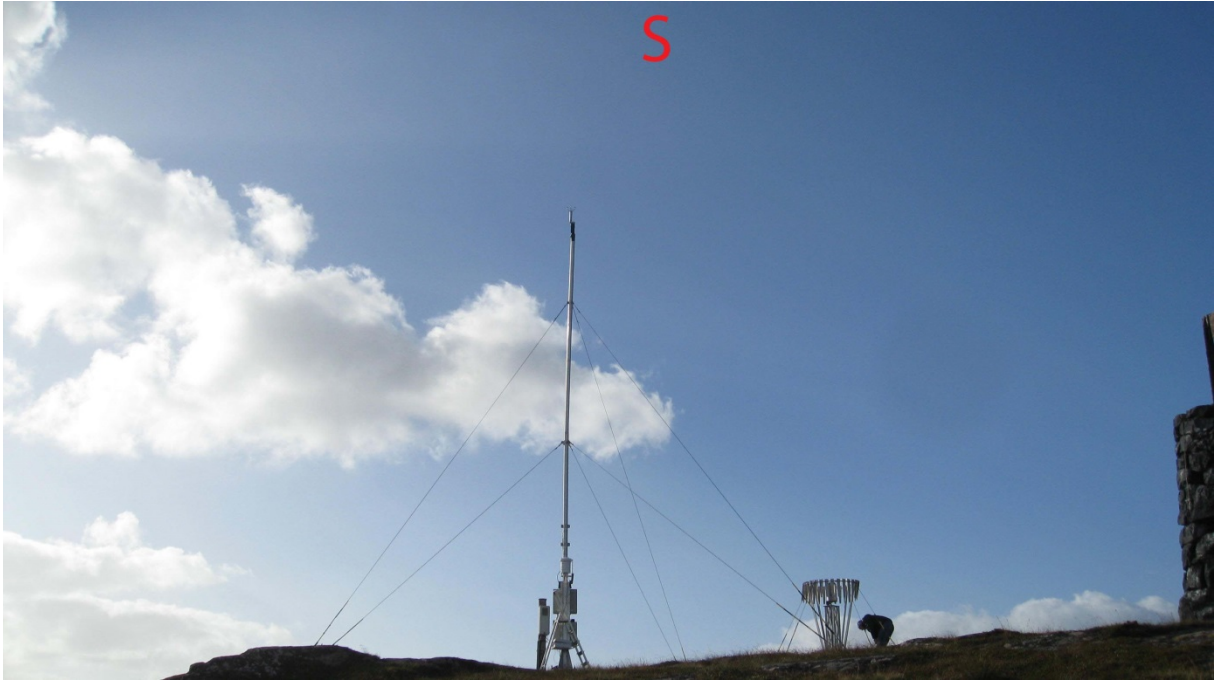
Weather station towards South
