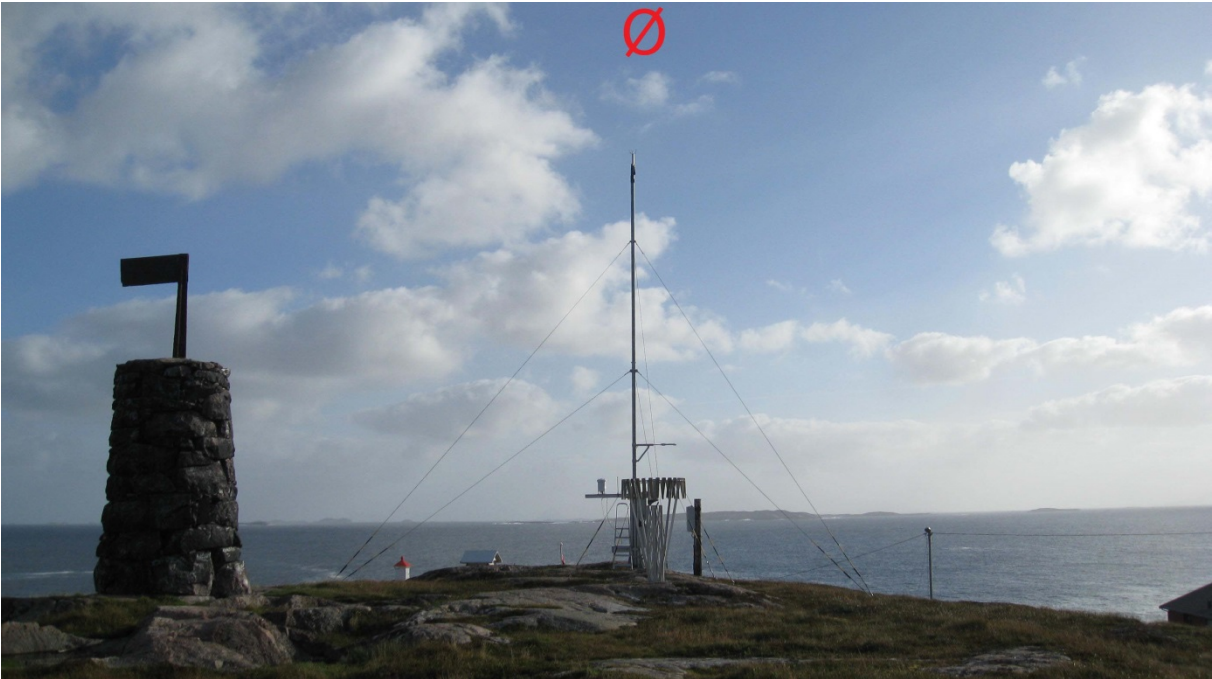
Weather station towards East
