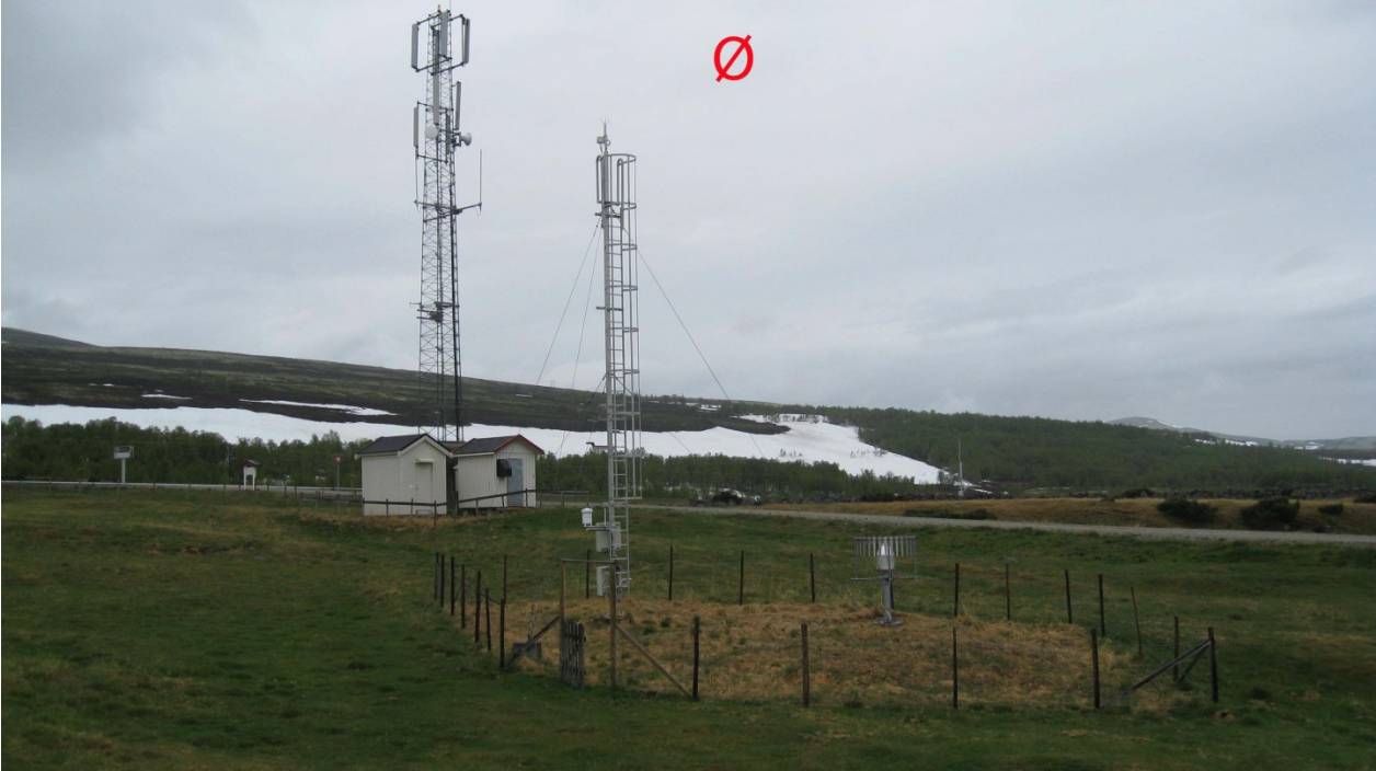
Weather station towards East
