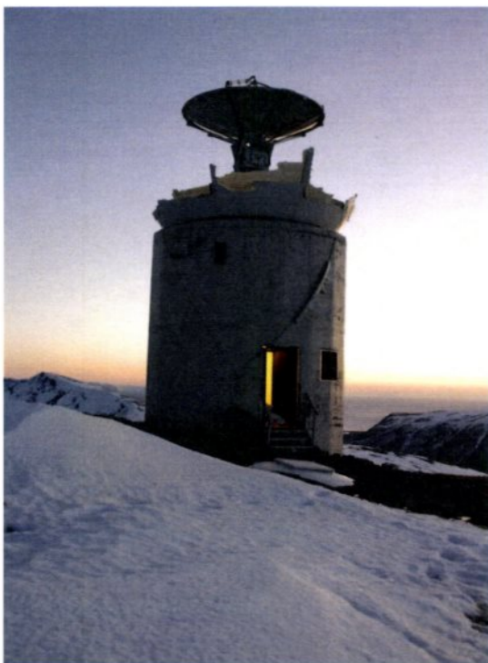
Figure 4 Antenna secured in 90 degrees angle
