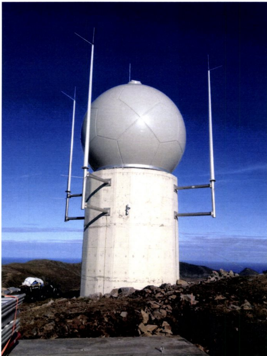
Figure 10. Picture of Andøya weather radar with the new lightning protection equipment.
